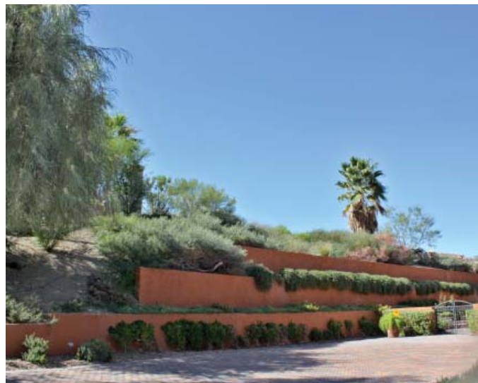
Terraced, site retaining walls and integrated planting help blend the development into the landscape.
