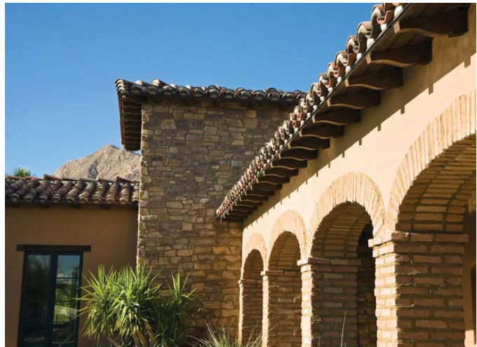
The blending of natural materials such as wood and stone helps to create a harmonious design.
