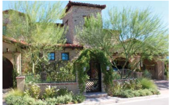
Courtyard and Courtyard Walls
