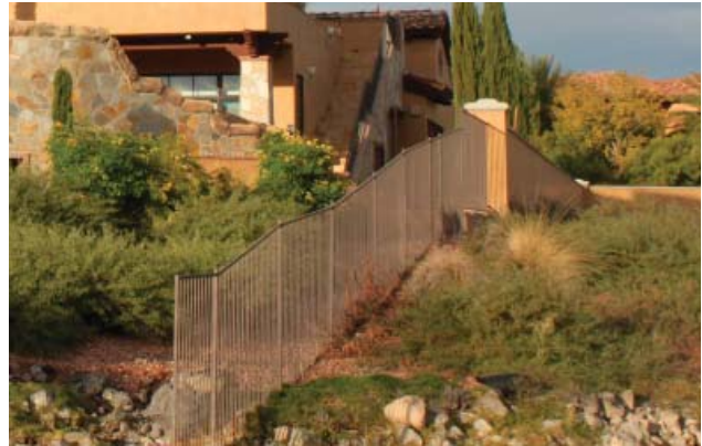
Typical property line wall and view fence
